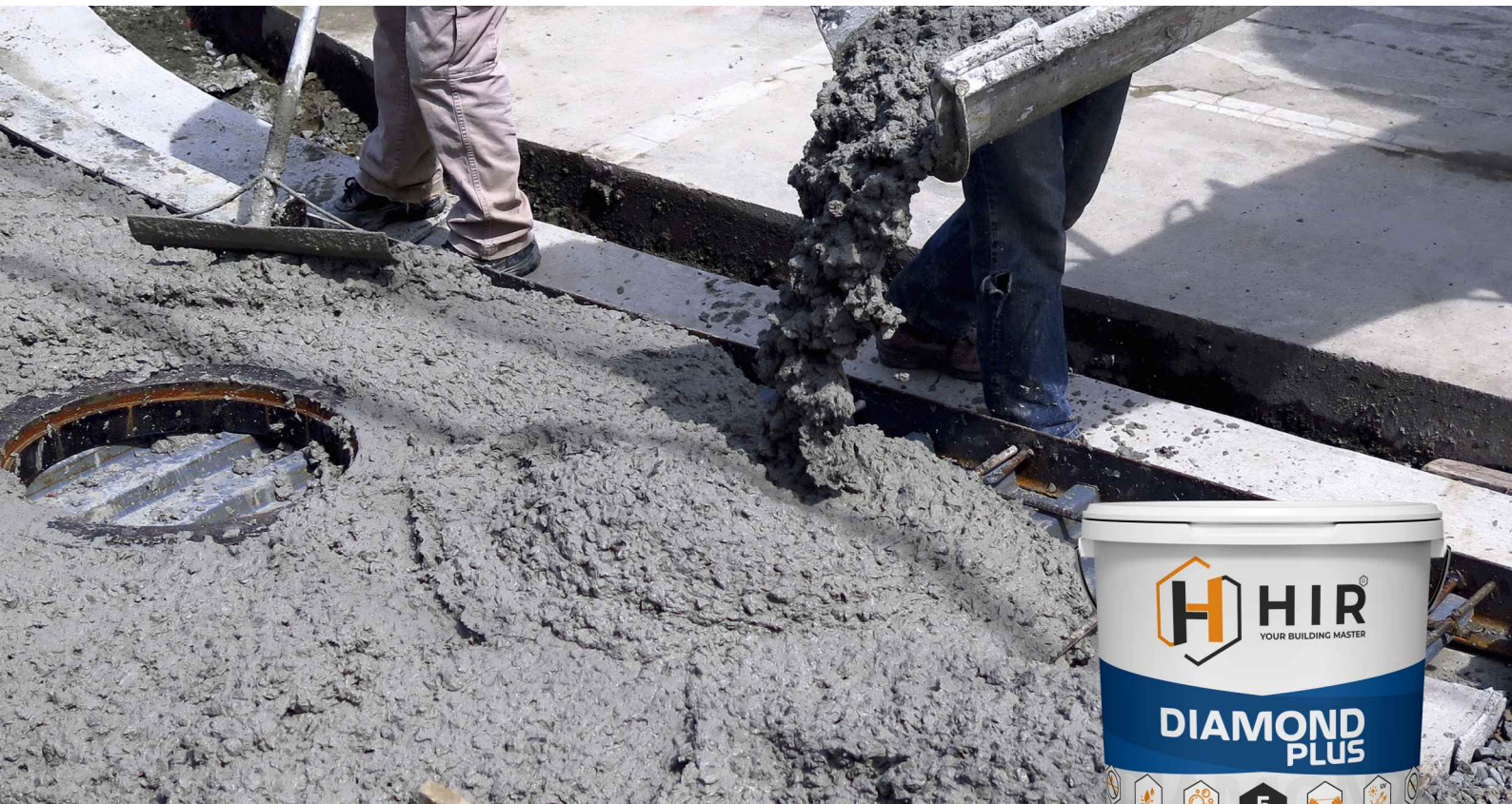
Concrete mixture machine/terrace/rcc building work
